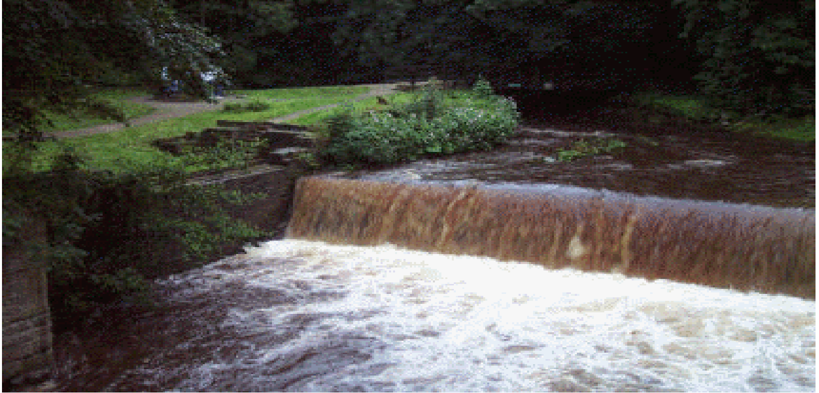
Figure 2 Torr Site in July 2007 after a day of heavy rain
